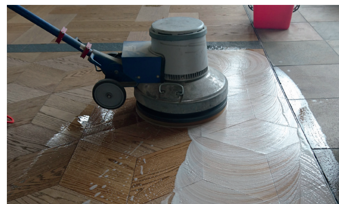
► Fig. 3 Rubbing with a polishing machine
